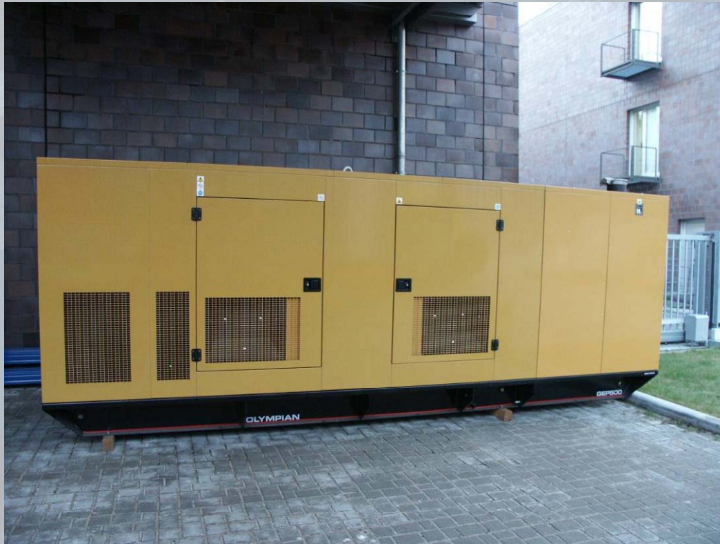
500 kVA Diesel Generator
